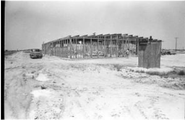
UFW Office Building under construction at Forty Acres
