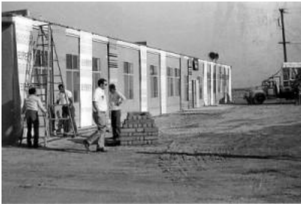
UFW Office Building nearing completion. 1969
